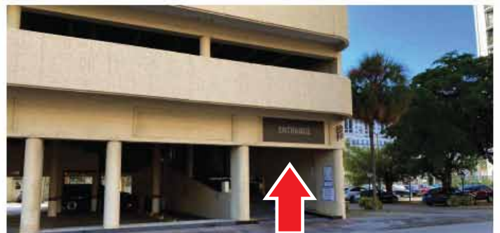
RAMP ACCESS PARKING GARAGE
